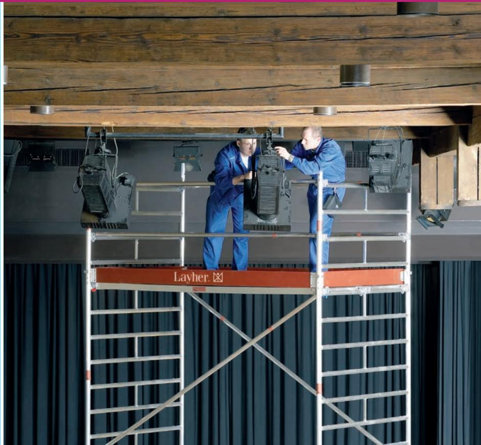
**The universal tower with double-width working surface provides a comfortable workplace at great heights.**
